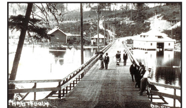
Open Span Chautauqua Bridge
